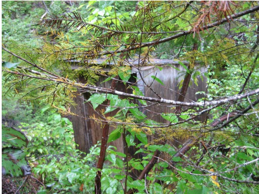
Shelter room at water outfall (Site Visit -1)
