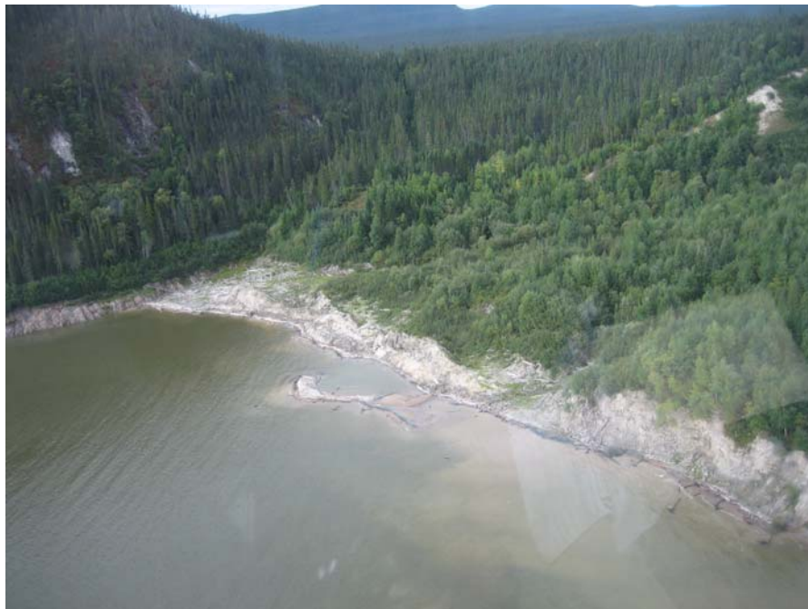
Downstream slope (Site Visit -1)
