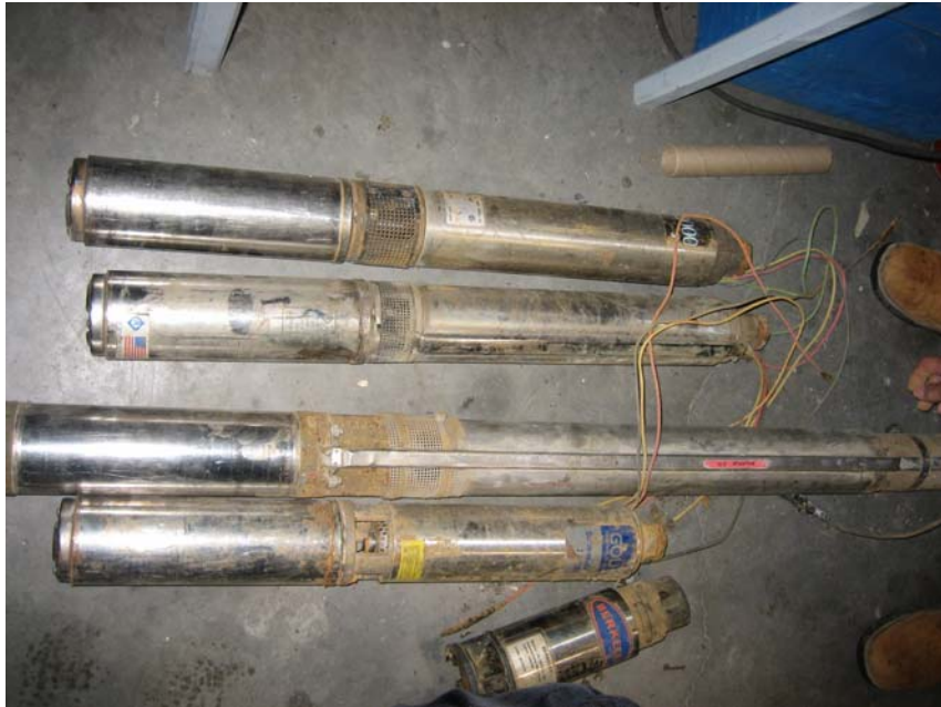
Decommissioned pumps (Site Visit -1)
