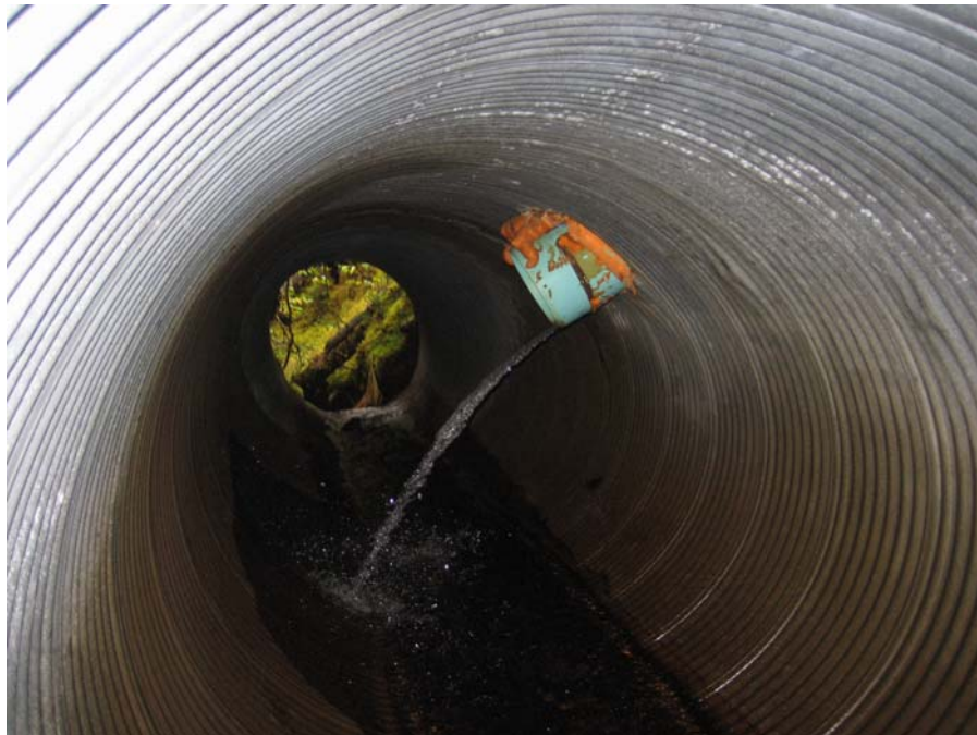
Discharge water from outfall pipe (Site Visit -1)
