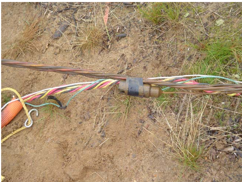
Level Electrode removed from W4 (Site Visit -1)
