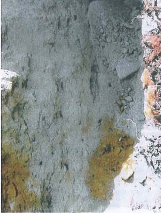
Test pit excavation
