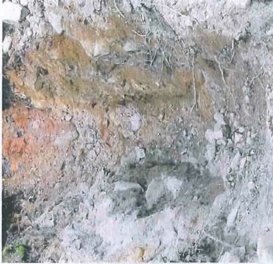
Test pit excavation
