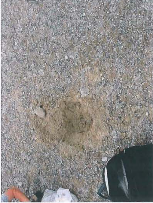
Hand dug excavation
