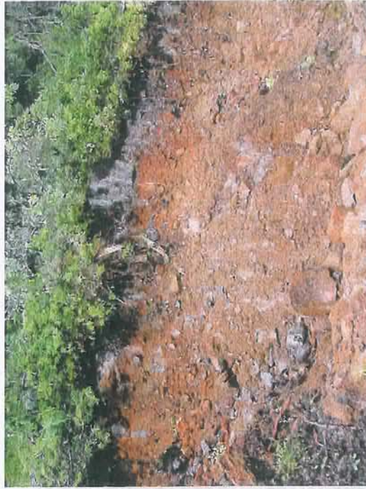
Test pit excavation - View 1
