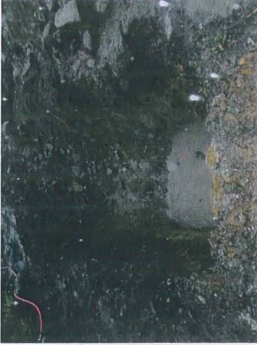
Test pit excavation
