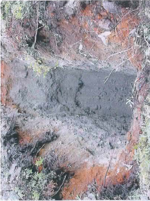
Test pit excavation
