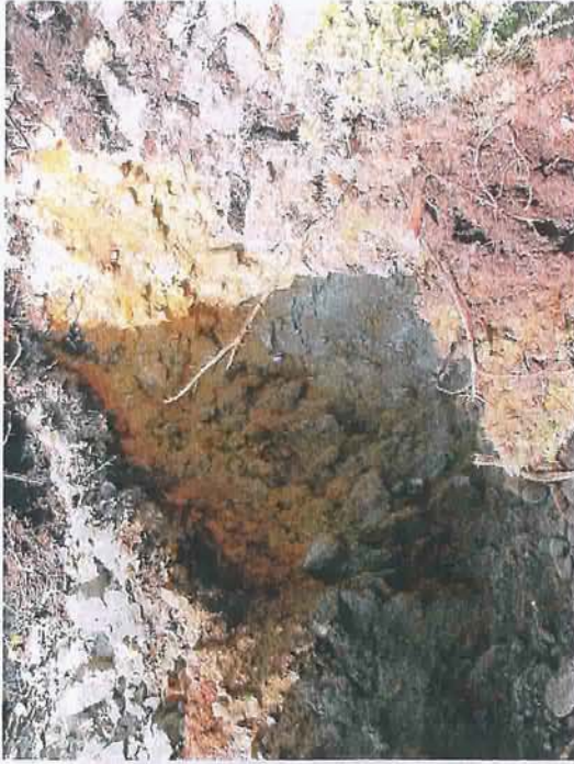
Test pit excavation
