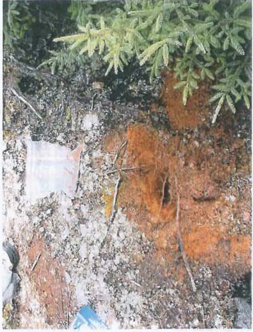
Hand dug excavation
