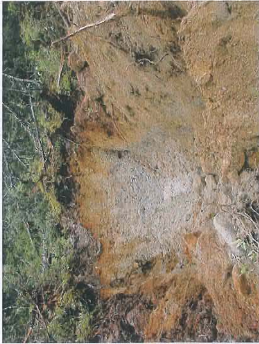
Test pit excavation
