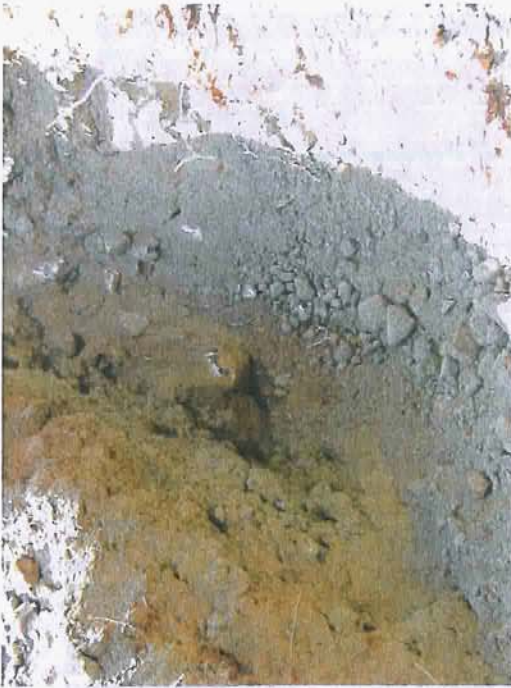
Test pit excavation
