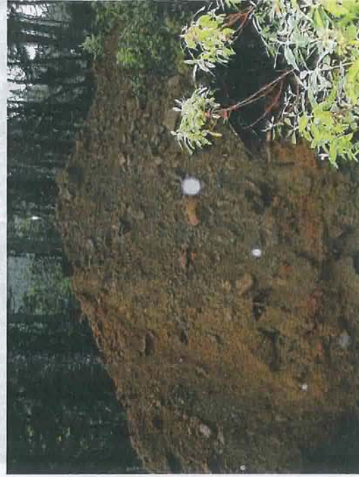
Spoilage from the test pit excavation
