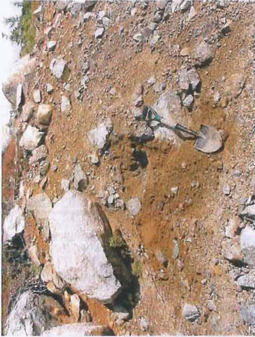
Hand dug excavation
