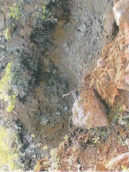
Test pit excavation
