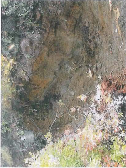
Test pit excavation
