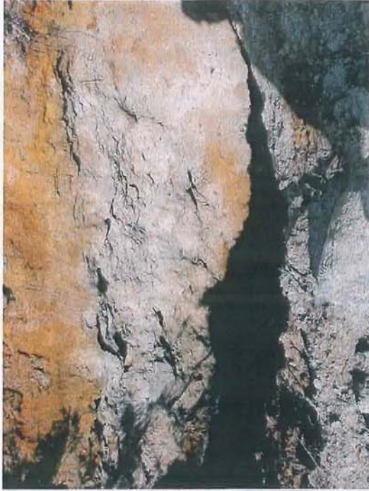
Test pit excavation
