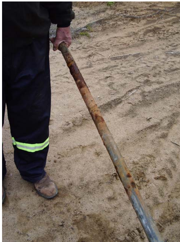
Photograph 4: The risers were inspected for corrosion and replaced as required.
