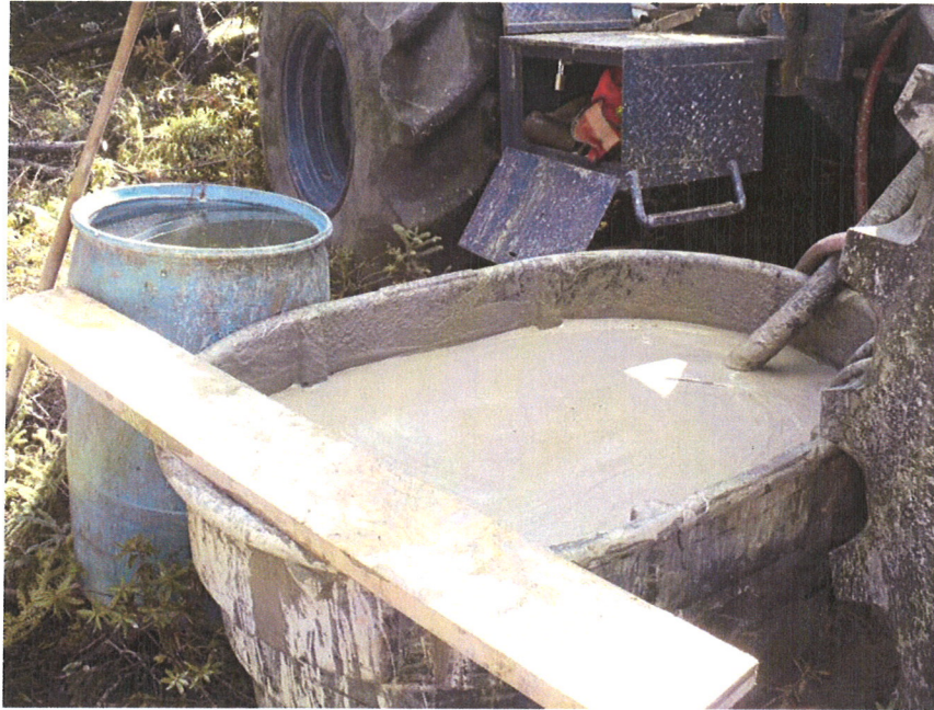
Photo 7 Mixing Grout 2009 P3
