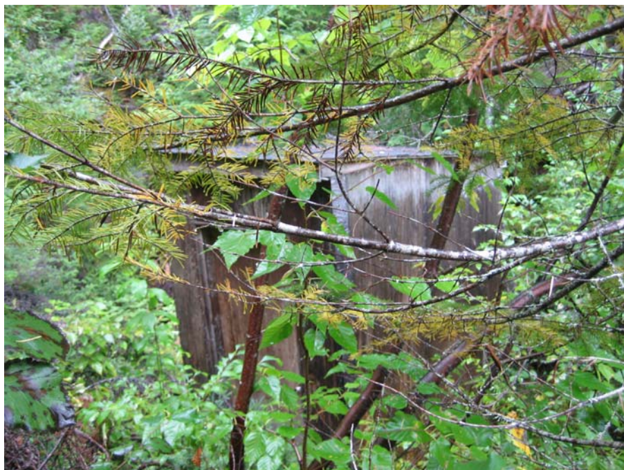
Shelter room at water outfall (Site Visit -1)
