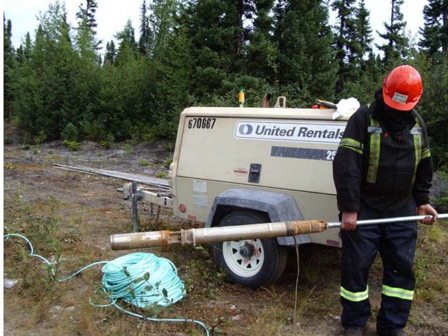
Photograph 5: The pump was inspected, the screen removed and all cleaned.
