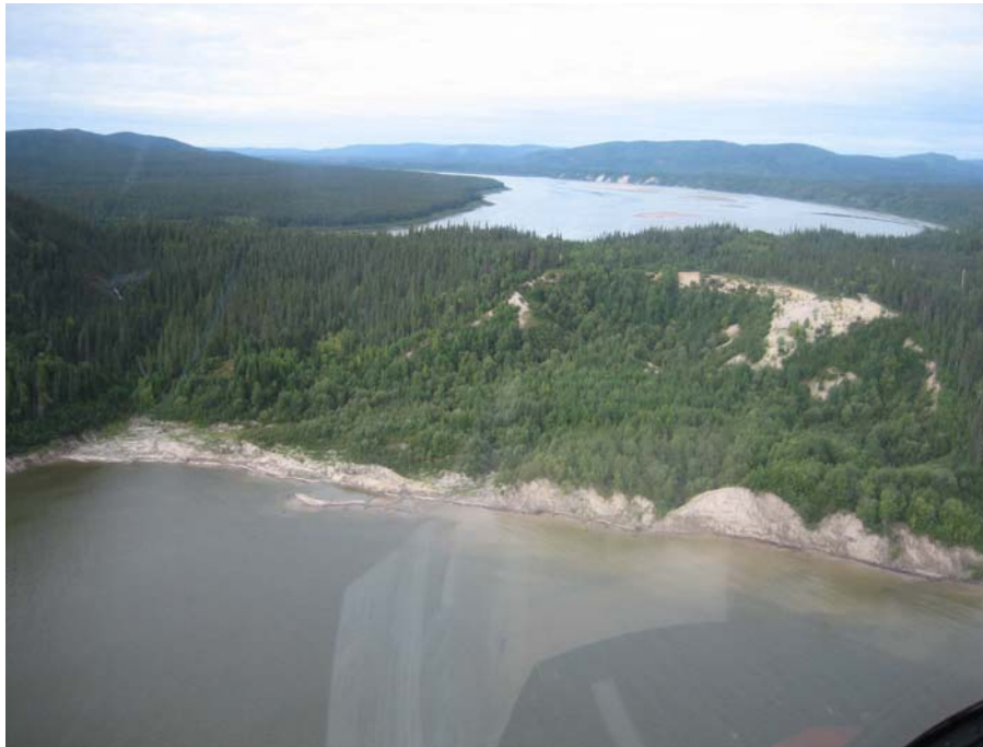
Downstream slope (Site Visit -1)
