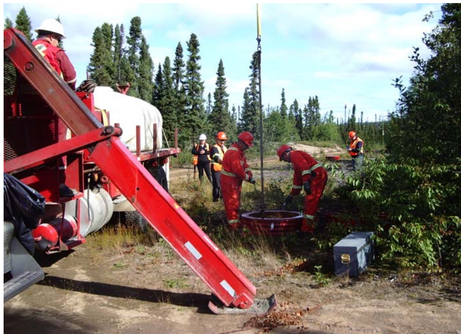
Photograph 2: The risers, wiring and pump were removed from each well.
