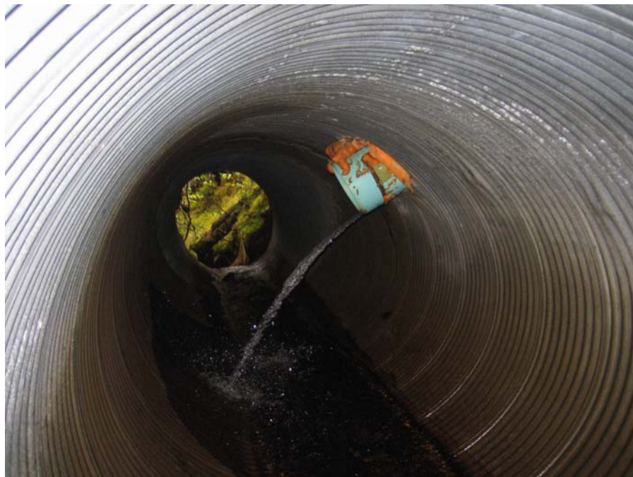
Discharge water from outfall pipe (Site Visit -1)
