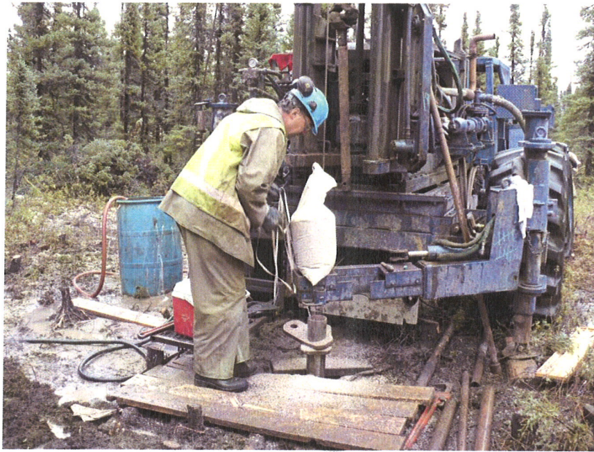
Photo 5 Well Install P4 (B)
