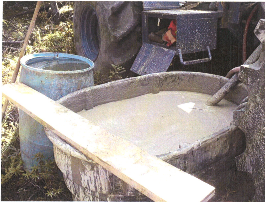
Photo 7 Mixing Grout 2009 P3
