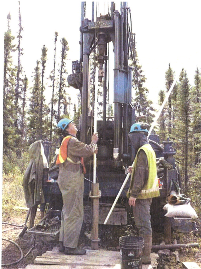
Photo 6 Well Install P4 (A)
