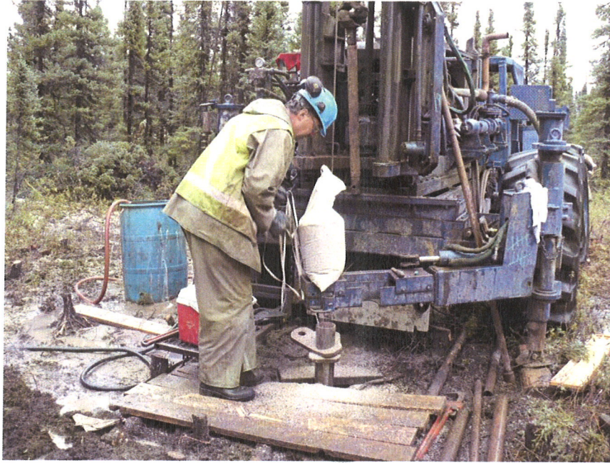
Photo 5 Well Install P4 (B)
