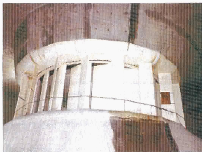
Figure 3-12: Example of a Semi-Frontal Scroll Case showing Phase 1 Concrete Walls and the Stay Ring Foundation
