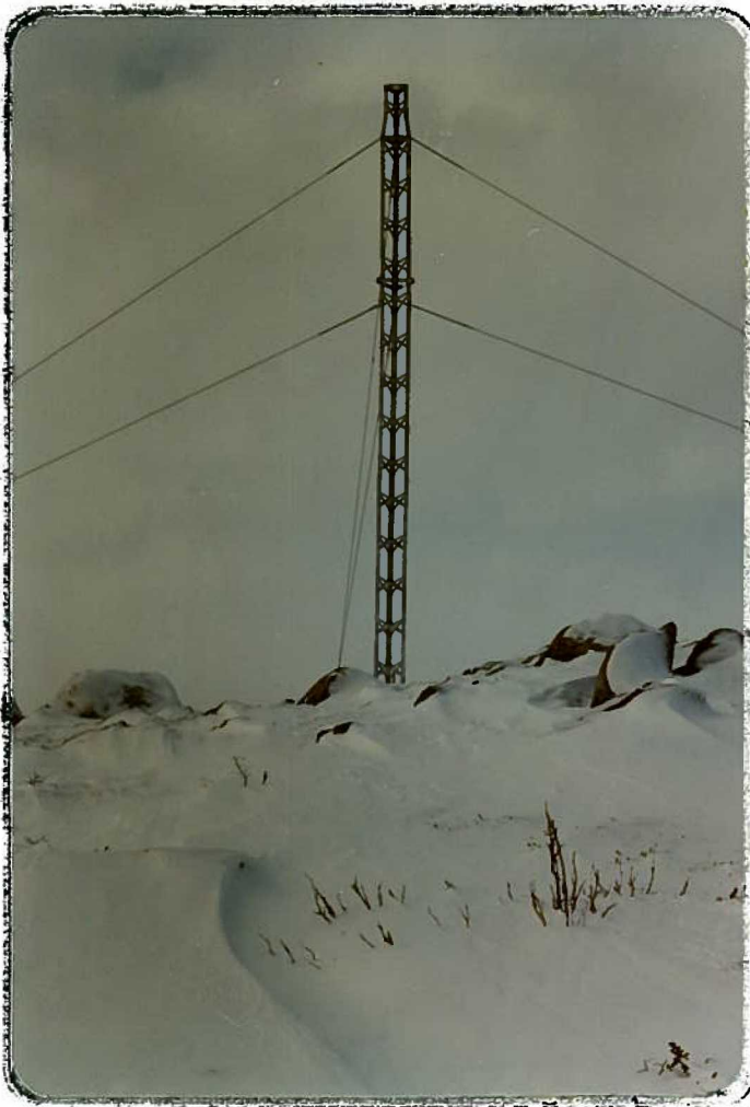
Photo V - New Test Site
