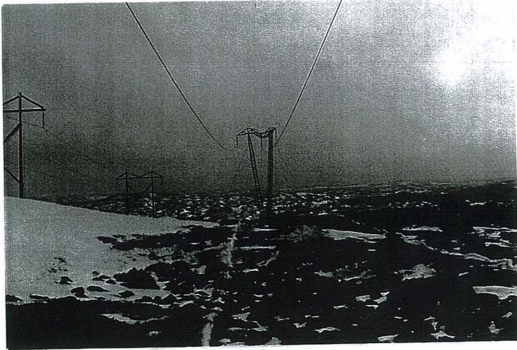
Photo No. 2-3 April 1988 Failure of bridge on Suspension Tower (TL-217) at Hawke Hill
