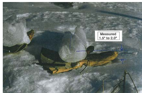
Fig. 5 Glaze ice observed during 1994 line failure
