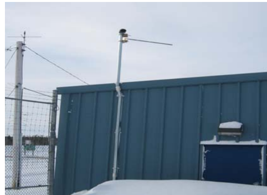
Fig. 19 RIGD beam installed at a terminal station
