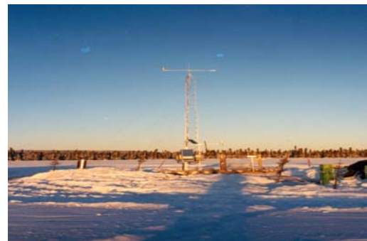
Fig. 15 Typical test tower installed at the Gull Island site (Labrador, Figure 1)
