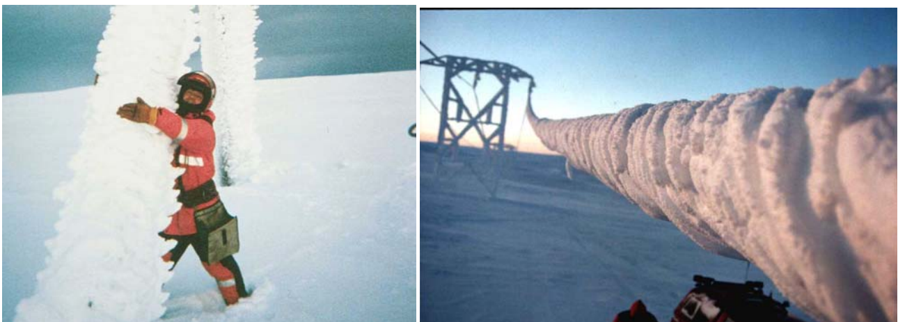
Figure 23. In-cloud icing on a guy wire.
