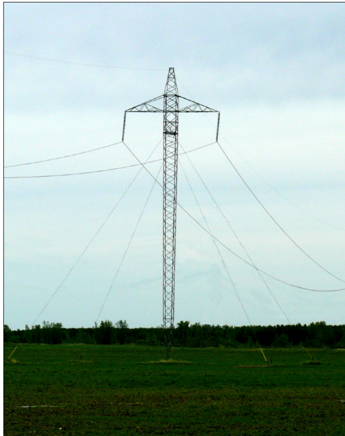
Figure 38. A typical tower in a HVdc line. Structurally the transmission line will be similar to other transmission lines in Newfoundland and Labrador and elsewhere.
