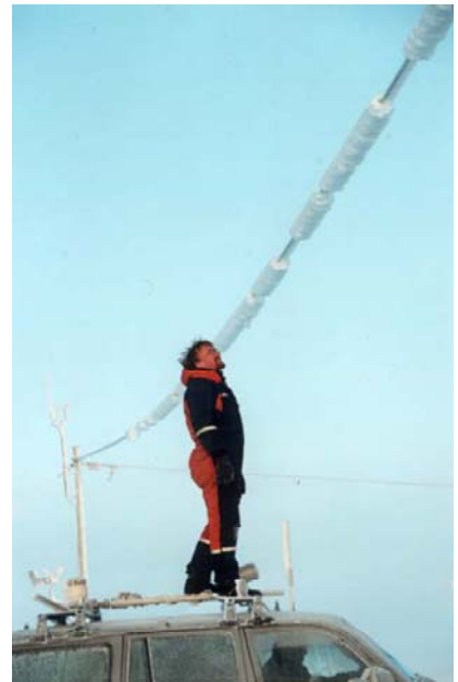
Figure 26. Icing in a test span (80m)
