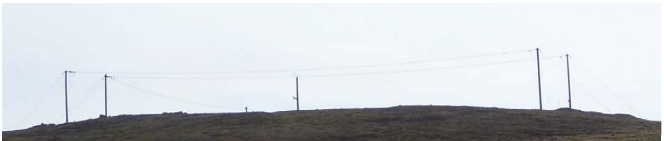
Figure 27. Test spans (3 spans) at Hallormsstadarhals (83-1).
